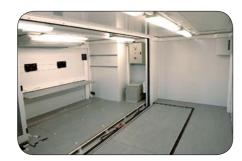
This upper deck container system is used for monitoring shipping traffic at sea and in ports. To protect the sensitive electronics in the two containers, a portion of the floor is equipped with shock absorbers. Power is supplied by a transformer that is integrated in the floor.
