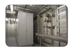
Furthermore, the containers were fitted with a double floor, cable lines and foundations for the technical equipment. The containers were also equipped with removable side walls to make future maintenance easier.
